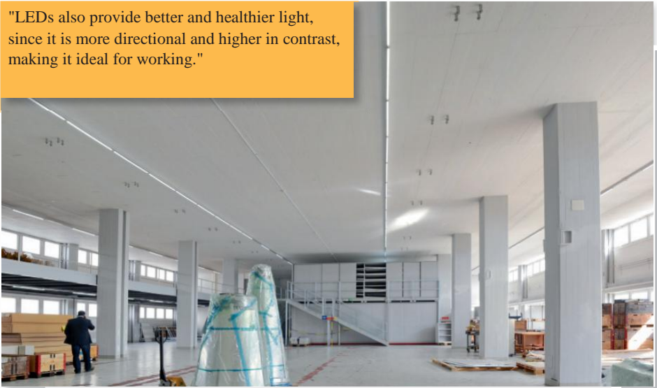
In the warehouse: Here one has a good view of the four LED tube strands, which allow homogeneous, flicker-free illumination of the room at the push of a button.
