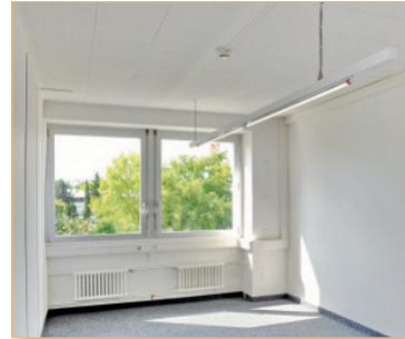
View of a conference room: Here, existing busbars were simply converted, with the corresponding adapters the LED tubes could be used, saving tremendous costs: Functionality and simplicity for good light.
